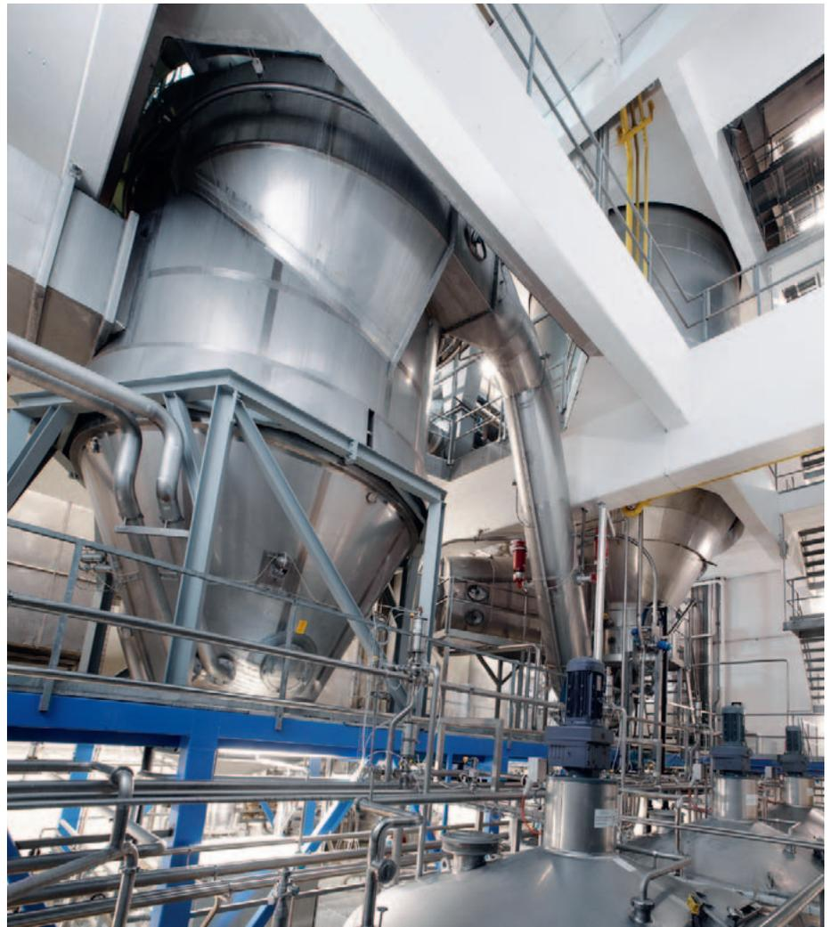
Spray dryer at Nutritec AG: energy savings thanks to comprehensive analysis using Pinch technology
